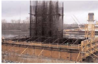
The I-895 Pocahontas Parkway crossing, with massive footings and columns exceeding 16 ft thick, maintained thermal mass concrete specifications and exceeded 5,000 psi 28-day design strengths using a 75 percent slag cement mixture.
