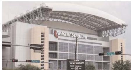
The four "super columns" supporting the retractable roof at Houston's Reliant Stadium consistently achieved field strengths of over 15,000 psi, yet maintained a strict temperature differential and peak temperature, using a portland-slag cement-fly ash mixture.
