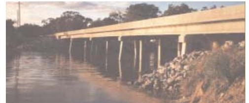
*The Charenton Canal Bridge, Louisiana's first HPC bridge deck, achieved a chloride permeability of less than 2,000 coulombs, using a 50/50 percent portland-slag cement mixture.*
