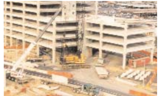
Precast/prestressed elements at the Philadelphia Airport parking garage incorporating slag cement.
