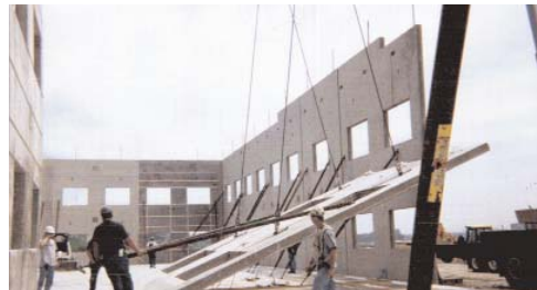
Precast tilt-up elements incorporating slag cement are made on the jobsite.
