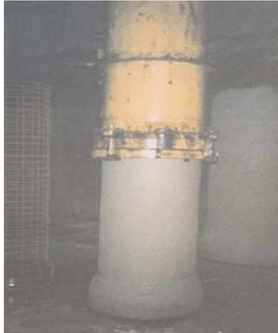
Concrete pipe manufactured with slag cement.
