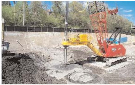
Figure 1 - Brownfield Remediation at WE Energies site in Appleton, WI
