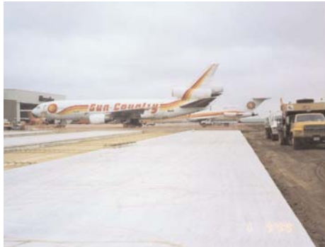
In 1998, airfield pavements were constructed at the Minneapolis Airport using a portland blast-furnace slag blended cement consisting of 35% slag cement, with an addition of 10% Class C fly ash. Performance of the concrete has been excellent.
