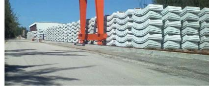
*Figure 3 Precast segments used in Port of Miami Tunnel.*
