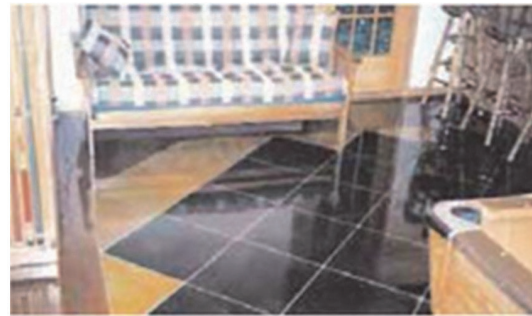
Self-consolidating concrete for residential floor slab using 50% slag cement, 50% portland cement.
