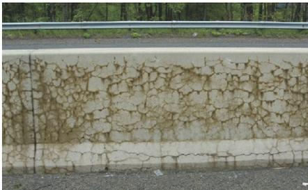
Figure 1: ASR causes expansion and cracking of concrete structures and pavements.
