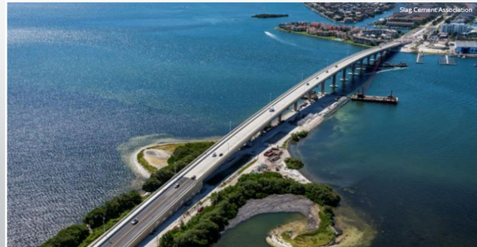
SR 679 Pinellas Bayway Bridge
