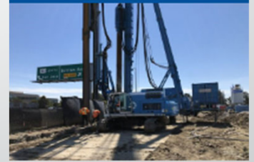
Slurry Cutoff Walls
