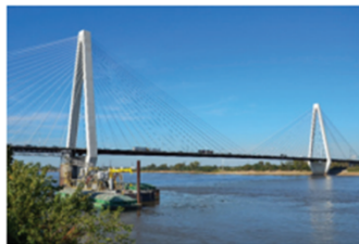
Figure 1: The I-70 Stan Musial Veterans Memorial Bridge (opened 2014) pylons used 70% slag cement in the mass concrete mix, which also was used in other concrete classes of the structures
