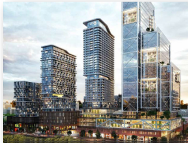
Ellis Don - The Well Mixed Use Development, Spadina & Front, Toronto 60,000m 3
