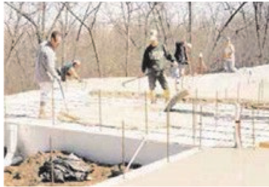
Self-consolidating concrete for residential floor slab using 50% slag cement, 50% portland cement.
