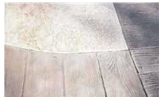
Decorative residential concrete with 25% slag cement: Interior acid stained concrete (top) and exterior stamped and colored concrete (bottom).
