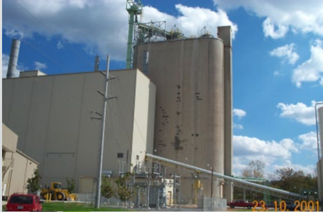
Slag cement plant
