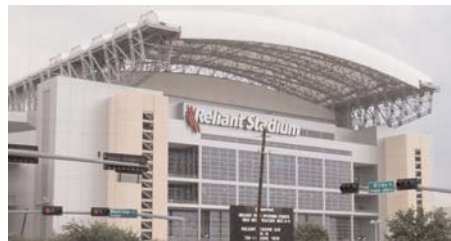
The four "super columns" supporting the retractable roof at Houston's Reliant Stadium consistently achieved field strengths of over 15,000 psi, yet maintained a strict temperature differential and peak temperature, using a portland-slag cement-fly ash mixture.
