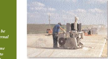
Joints need to be cut before internal stresses in the concrete become great enough to initiate a crack.
