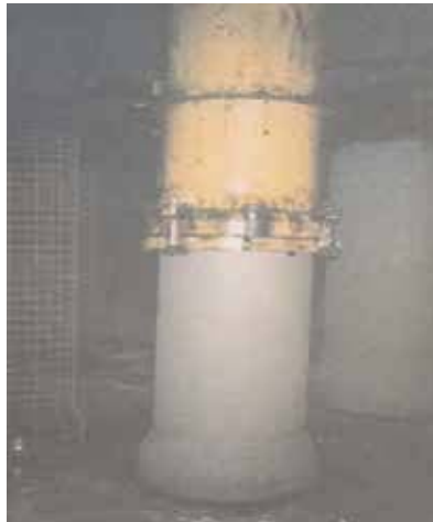
Concrete pipe manufactured with slag cement.
