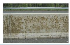
Figure 1: ASR causes expansion and cracking of concrete structures and pavements.
