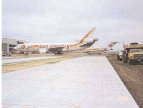
In 1998, airfield pavements were constructed at the Minneapolis Airport using a portland blast-furnace slag blended cement consisting of 35% slag cement, with an addition of 10% Class C fly ash. Performance of the concrete has been excellent.
