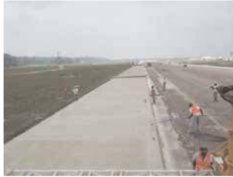
Airport paving at Spirit of St. Louis Airport in Chesterfield, MO, placed with blended cement (Type I (SM)) and Class C Fly Ash added separately.
