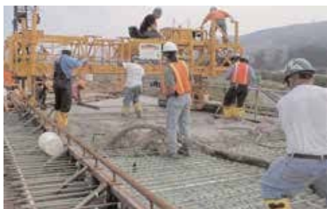
Figure 2: Route 64 bridge deck in Smithburg, MD used high performance concrete with 40 percent slag cement as part of a corrosion-resistant system that extended the predicted life of the structure by 37 years. (Contractor-Joseph Faye Co.; Concrete Supplier-Thomas Bennett Hunter)
